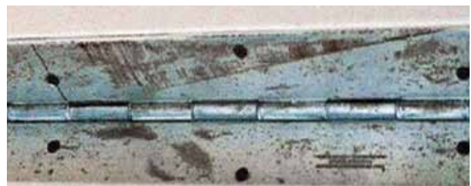
Figure 5: Carbon steel brushes were used by a cleaning contractor on this stainless steel door hinge that was installed beside an indoor swimming pool. The areas with carbon steel contamination are rusting. Photo courtesy of TMR Consulting
