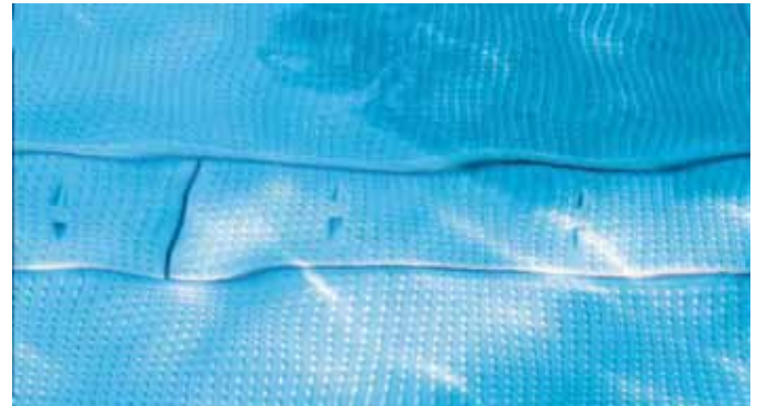
Figure 10 and 11: Type 316 pool gutters and water jet openings in the floor plates. Photos courtesy of Martina Helzel
