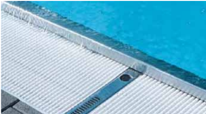
Figure 10 and 11: Type 316 pool gutters and water jet openings in the floor plates. Photos courtesy of Martina Helzel
