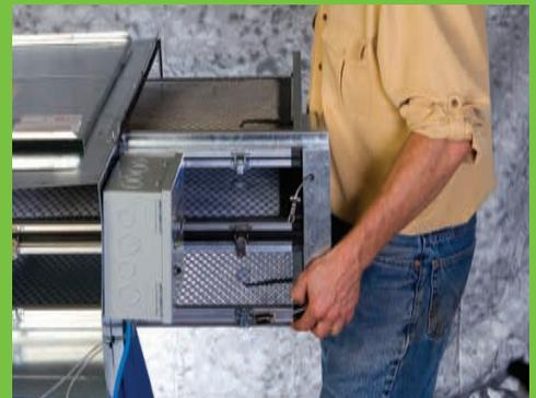
This is a slide out Dynamic V8 module in a filter box for a fan coil unit. These give a MERV 13 option for smaller equipment in LEED projects. This module was part of those that were installed throughout the LEED EB renovation of ASHRAE headquarters.
